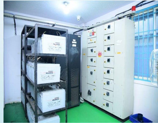
Installed UPS-160KVA
